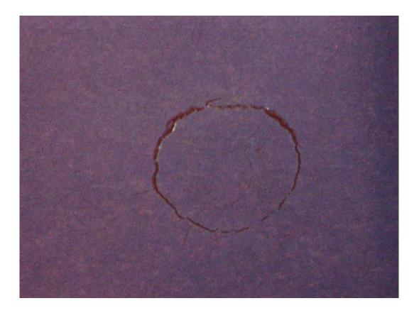
Cracking around the edges of a feather-edge repair.
