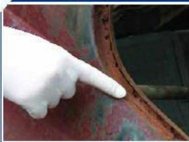
**BEFORE:** Rusted, leaking seam.
