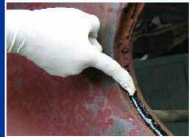
Press and contour bead into seam.
