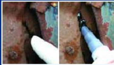
Fill in cracks in most surfaces.
